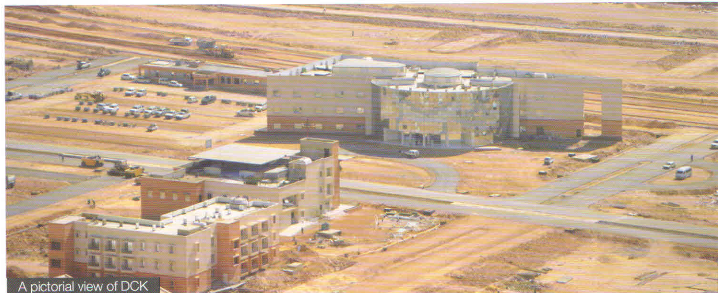
Another view of the fast paced development work
